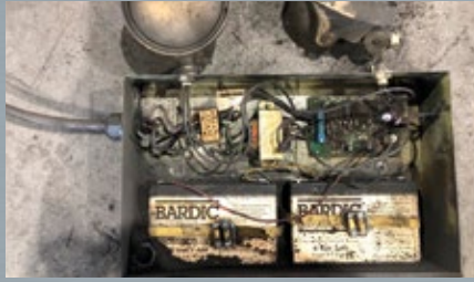
A broken safety light is a perfect example of a Paste Plant fire ignition source.
