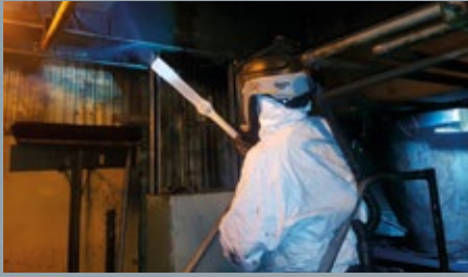
Cleaning the Paste Plant's walls with a dry ice pressure blaster.
